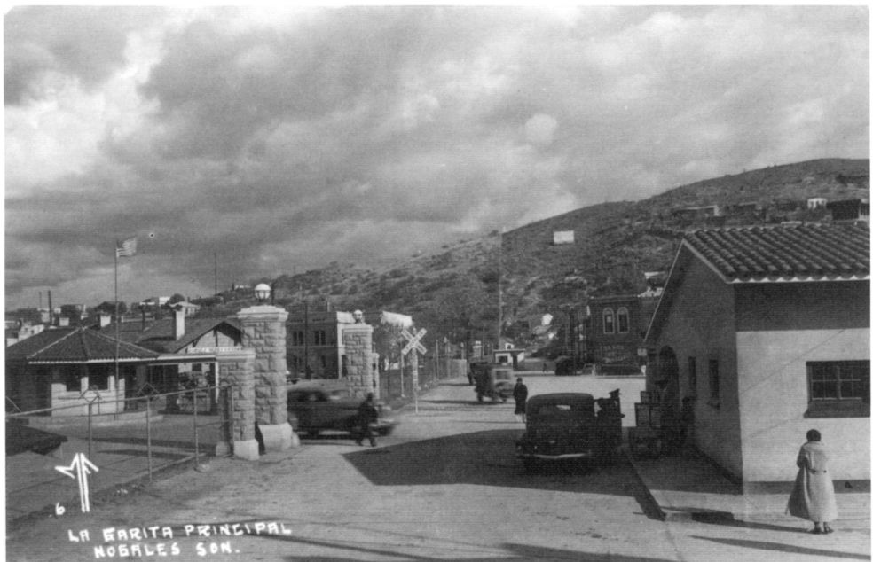
Figure 12. Main gate crossing, circa 1935. This unusual view looks east along the border fence from the main crossing with the back of the Mexican garita in the right foreground and the U.S. gatehouse in the left midground. The chain-link fence is seen extending over Chureas Hill in the far background. The Mexican garita at the Elías-Morley crossing is visible in the center midground.
