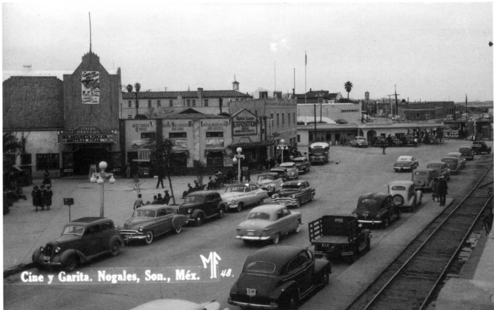
Figure 14. Main gate, circa 1952. The perspective is similar to that in figure 13, but the Mexican garita has been renovated into a single-story, flat-roofed, modern architectural style. A Safeway supermarket is now visible on the U.S. side. Many U.S. chain stores entered Nogales, Arizona, after World War II, and this Safeway store earned a reputation for high-volume sales because of the large number of Sonorans who would regularly shop across the border. On the Mexican side, the high art-deco facade facing Plaza Trece de Julio is the Teatro Obregón, featuring “Nuestras Vidas” on the marquee and “Gavilán Pollero” on the banner.
